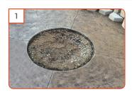
STEP 1 - Excavate your location for a drainstone base and fill excavated area with drain stone, level & compact.
